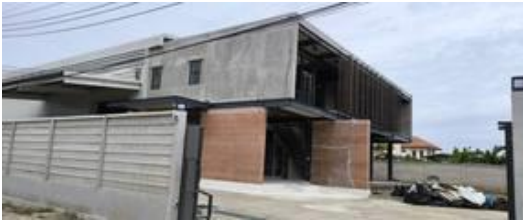
Case 01 · Warehouse + office
