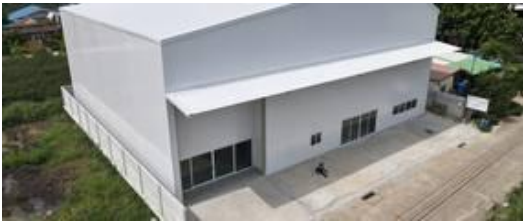
Case 04 · Distribution center B
