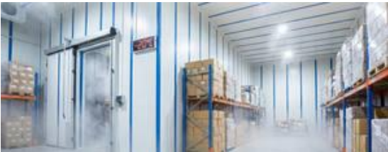
Cold storage Insulation, doors and energy efficiency
